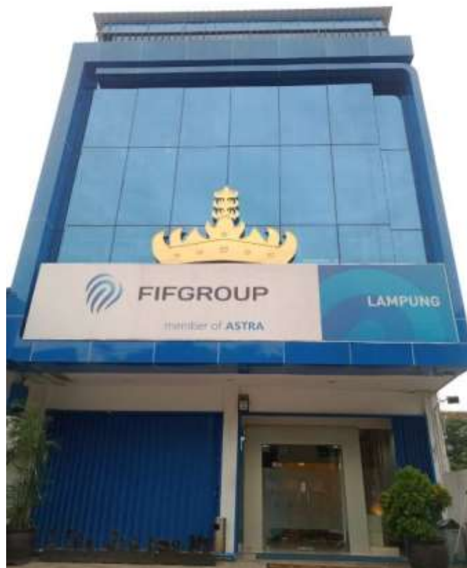
Gambar 3.3 Kantor Perusahaan PT Federal International Finance
