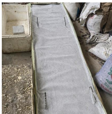
Gambar 3.35. Proses curing panel beton ringan.
