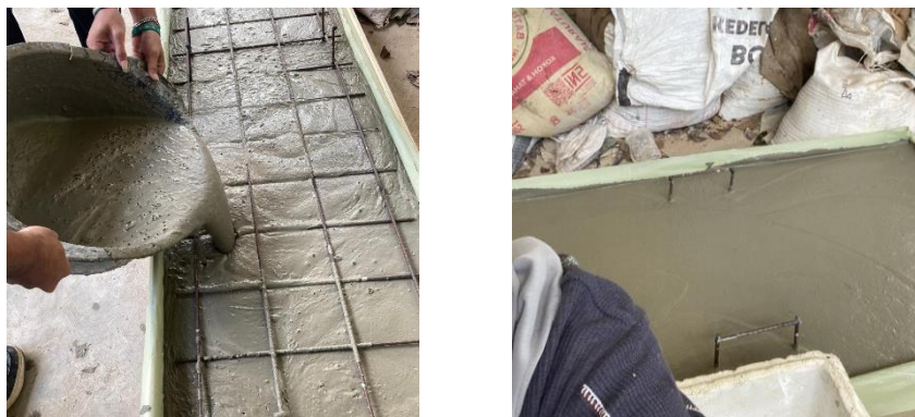
Gambar 3.35. Proses pengecoran panel beton ringan.
