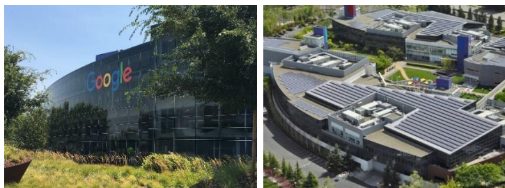
Gambar 2. 36 Googleplex Building Sumber : Google
