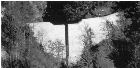
Gambar 7. Check Dam Tipe Slit
