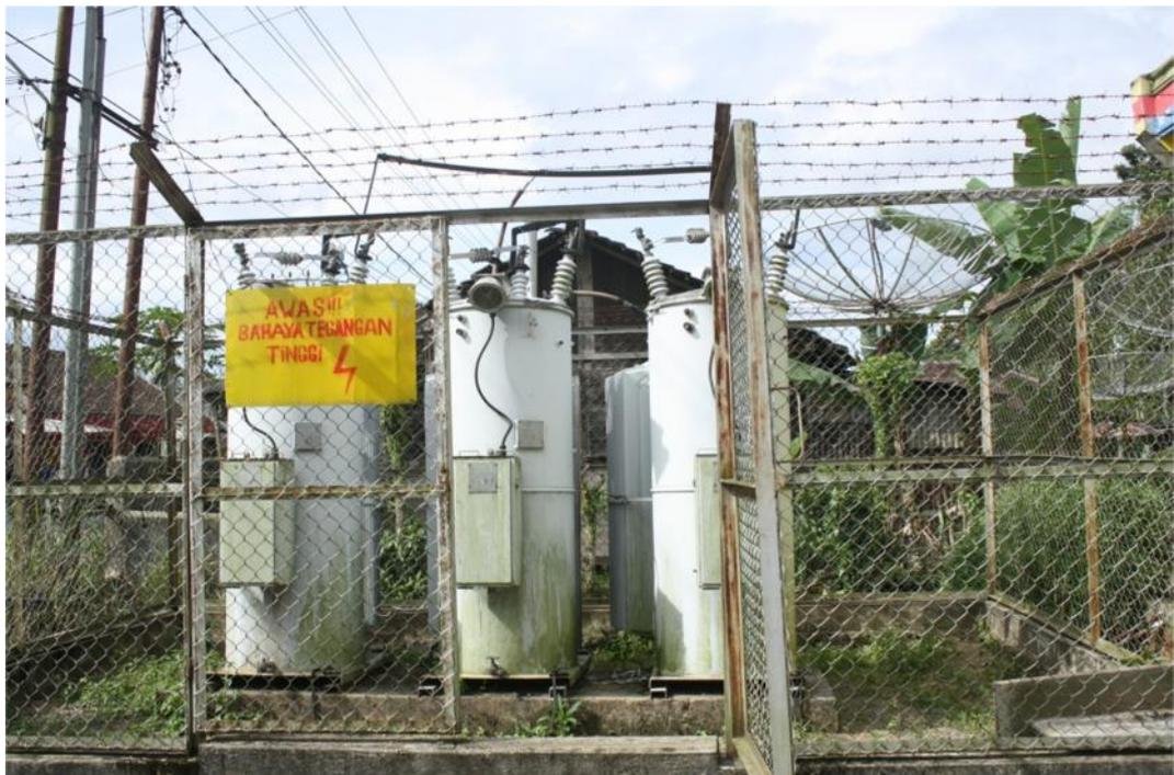
Gambar 2.1. *Step Voltage Regulator*
