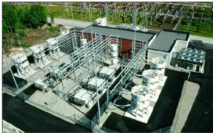
Gambar 2.3. Static Var Compensator[3]
