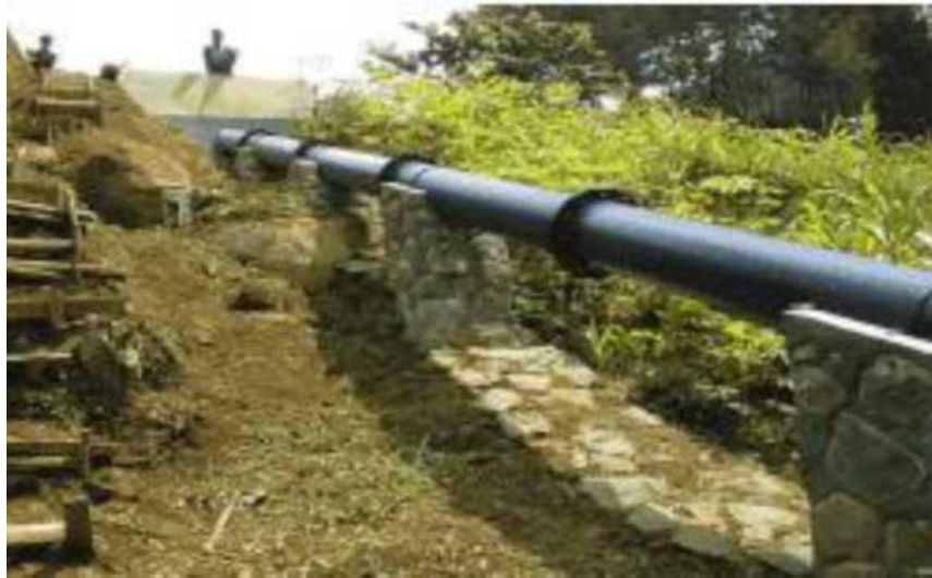
Gambar 2.6. Pipa pesat ( pen stock ) (Laymand, 1998).
