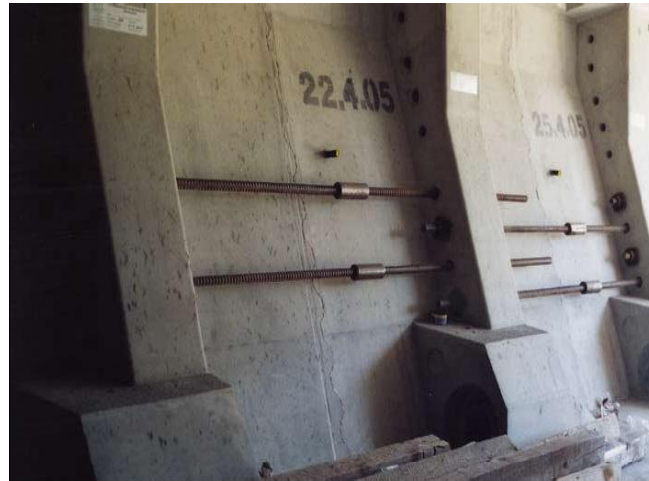
Gambar 2.5 Temporary tendon
