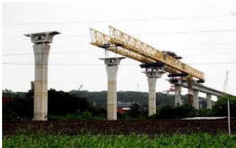
Gambar 2.13 Launching gantry
