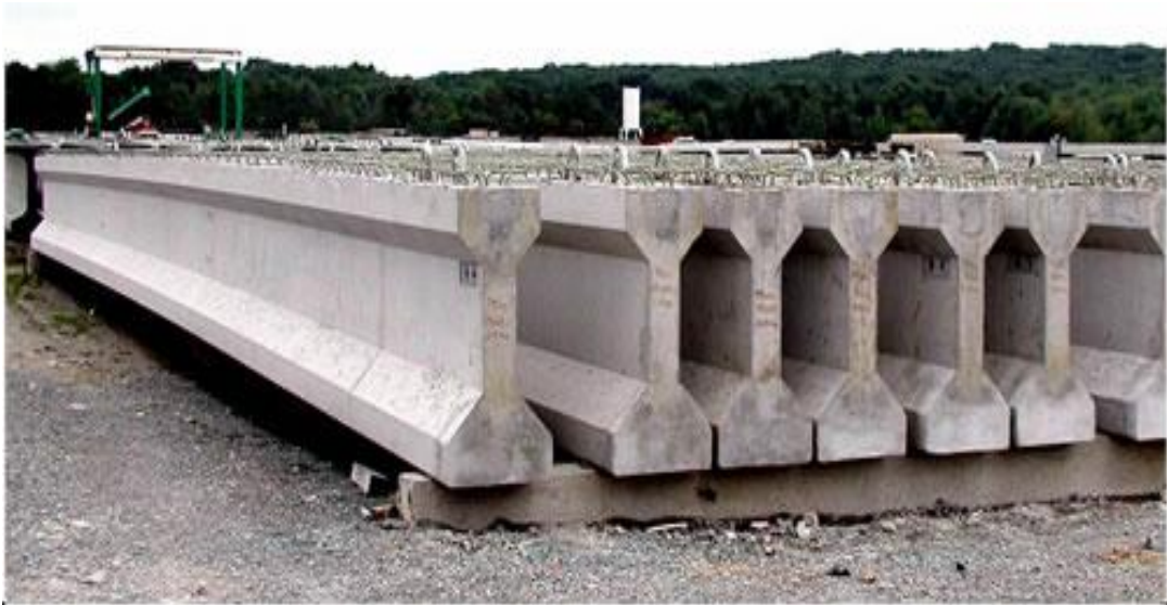
Gambar 2.8 PCI girder
