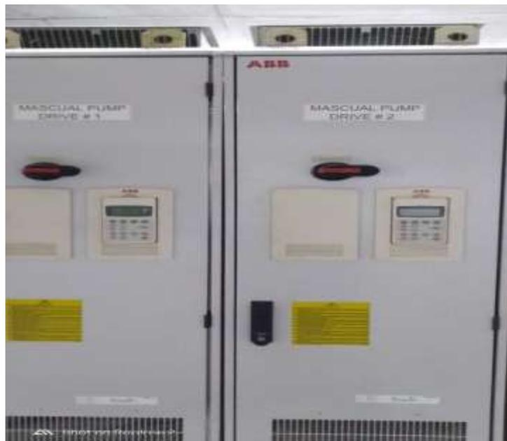
Gambar 2.9 Inverter ABB ACS800
