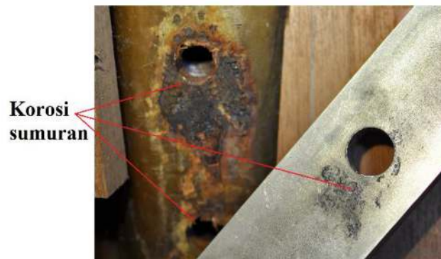
Gambar 2. Korosi sumuran (Cramer, 2003)
