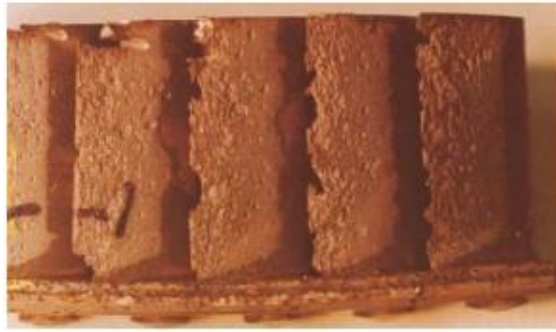
Gambar 7. Erosion/ abrasion corrosion
