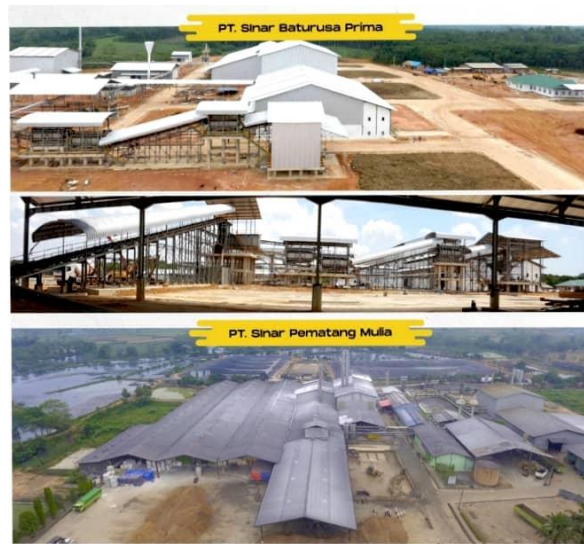
Gambar 6. Tapioca Starch Processing Plant
