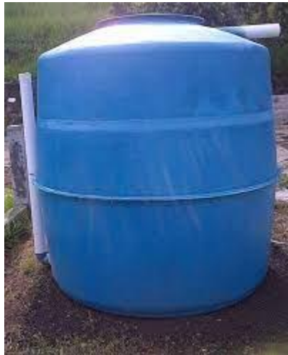
Gambar 6. Digester Tipe Fiberglass
