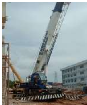
Gambar 3. 17 Mobile Crane (Derek Bergerak)
