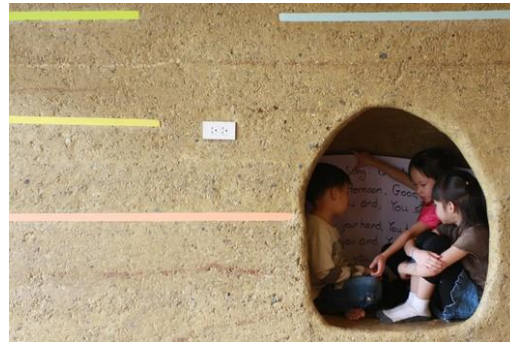
Gambar 2.14 Dinding Rammed Earth Sumber: archdaily.com
