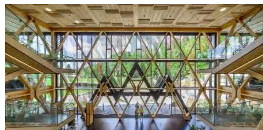
Gambar 2. 7 Sistem Diagrid
