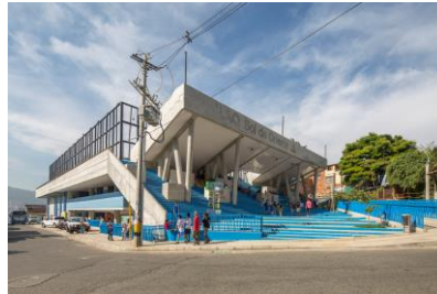
Gambar 2.15. UVA Sol De Oriente Community Center . Sumber: Diakses melalui www.archdaily.com , 18 Maret 2021
