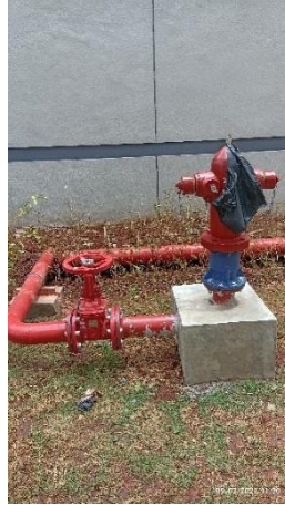
Gambar 3. 35 Hydrant Pilar
