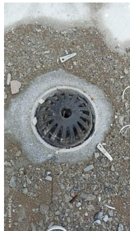
Gambar 3. 43 Roof Drain
