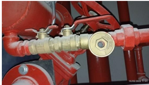
Gambar 3. 39 Sprinkler Flusing
