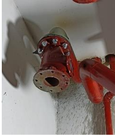
Gambar 3. 20 Flange Pipa
