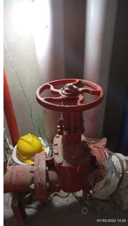
Gambar 3. 21 Get Valve Body Flanges Ends
