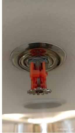
Gambar 3. 38 Head Sprinkler
