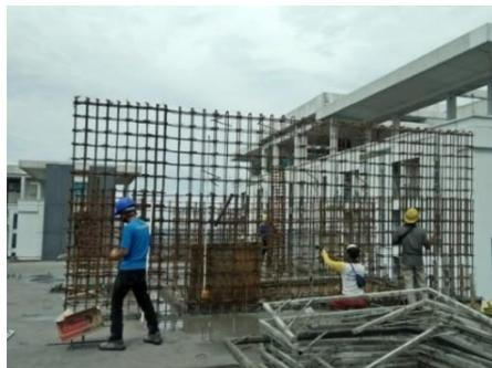
**Gambar 3.45** Penulangan *Shear Wall* Lantai 16
