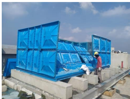
Gambar 3. 24 Roof Tank
