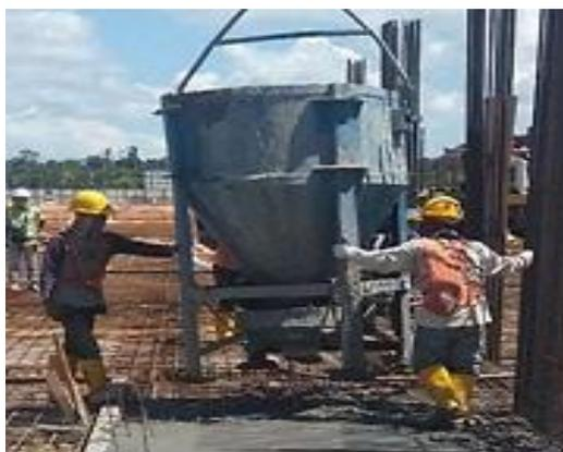
**Gambar 3.28.** *Concrete Bucket*
