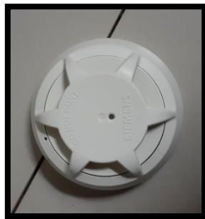
Gambar 3.34 Smoke Detector
