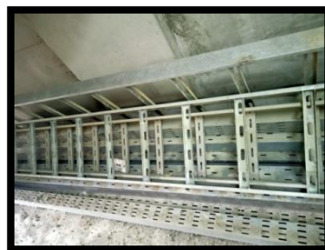
Gambar 3. 26 Cable ladder
