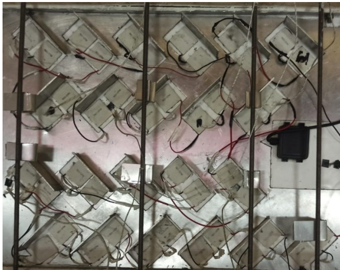
Gambar 3.18 Pemasangan TEC ( Thermoelectric Cooler )
