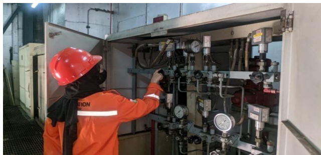
Gambar 3. 30 Survei Lapangan di Area Lube Oil System
