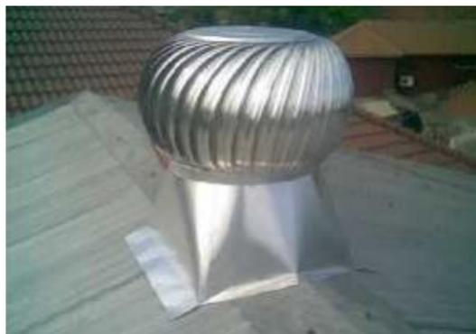
**Gambar 2.7** Turbin Ventilator *Cyclone* (Jamaludin, 2019)
