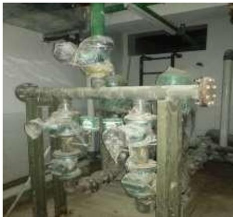
**Gambar 3. 19** pompa booster
