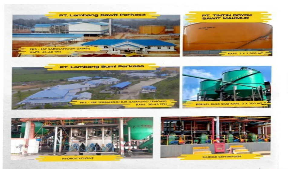
Gambar 5 Palm Oil Processing Plant Sumber : PT. Lambang Jaya 2023
