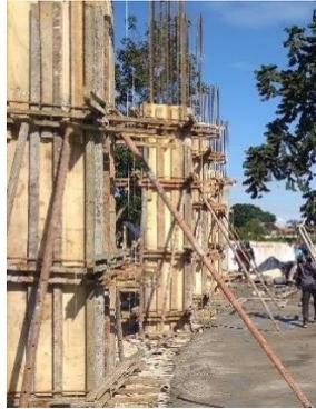
**Gambar 3.11.** Bekisting *Plywood*
