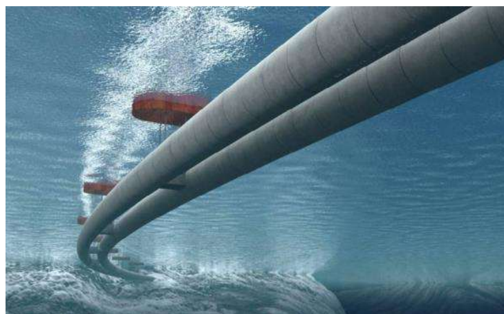
Gambar 2.2 Submerged floating twin tunnel
