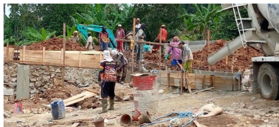
Gambar 3.8. Beton Ready Mix
