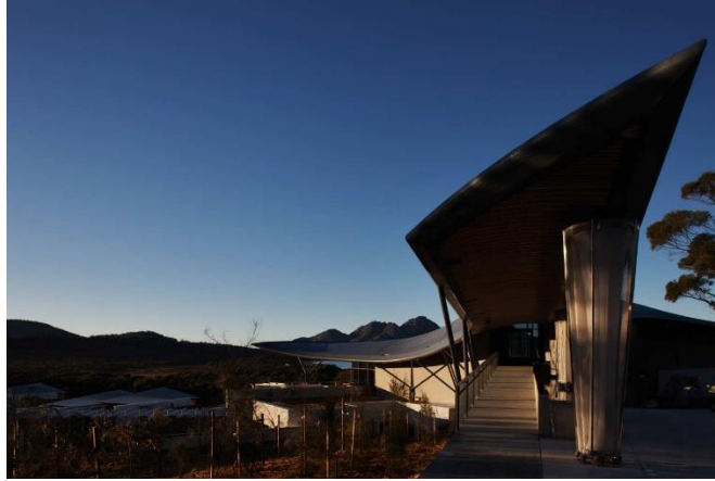
Gambar 2. 93 Entrance Saffire Freycinet Resort
