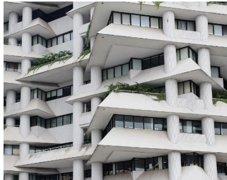
Gambar 2.24 Fasad Wisma Dharmala Sumber: hiddenarchitecture.net
