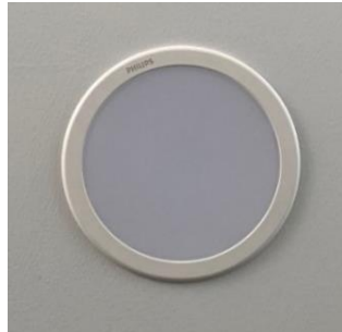
Gambar 3.8 Down Light LED (Sumber : Dokumentasi Pribadi)
