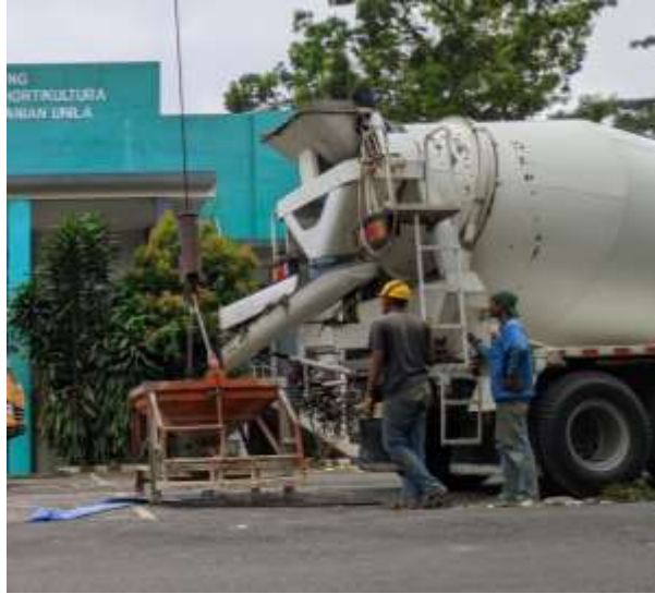
Gambar 3.11 Truk Pencampuran Beton (Mixer Truck Concrete)
