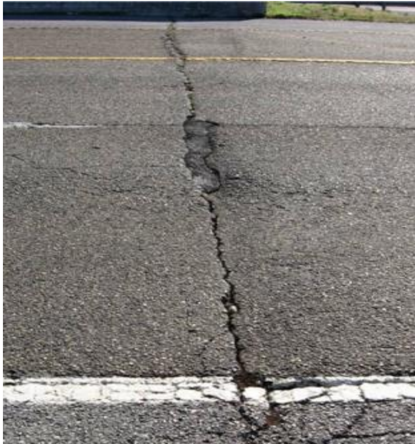
Gambar 4. Transversal Crack (Khare et al. , 2023)
