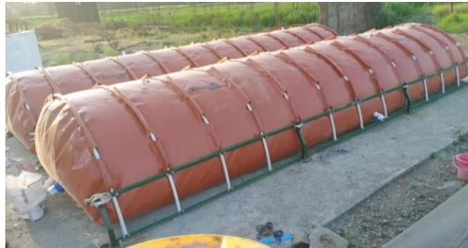
Gambar 4. Digester jenis *ballon plant* (Bodhe *et al.*, 2023)
