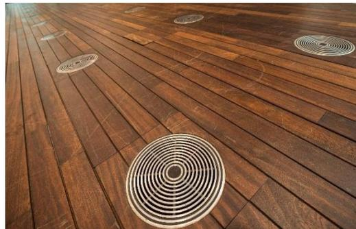
Gambar 2 65 Underfloor Air Supply
