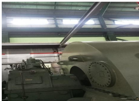
Gambar 2.16 Turning Gear
