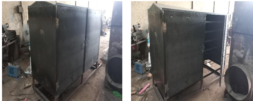
Gambar 3.6 Finishing Penempelan Dinding Bed Dryer
