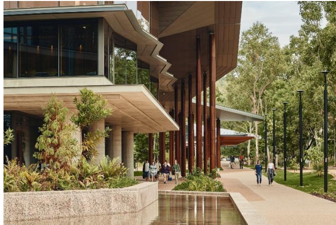
Gambar 2.27 James Cook University Engineering & Innovation Sumber: Archdaily
