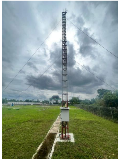
Gambar 2. 12 Struktur Automatic Weather Station (AWS).
